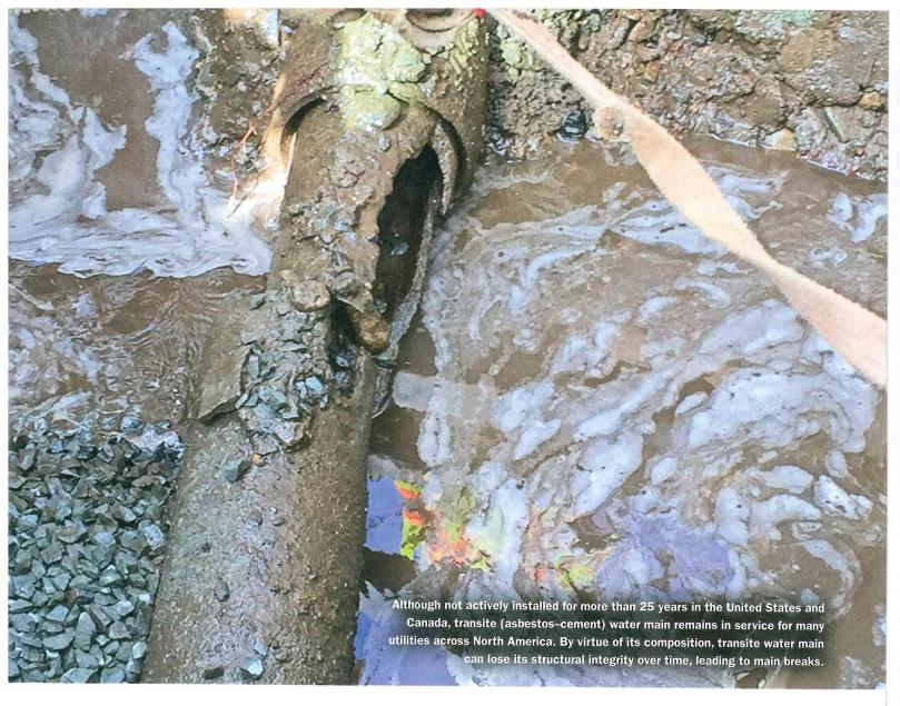
Fortunately, the main was isolated quickly. This minimized water loss from the break, but not before caverns undermining the street's integrity were created. The responding crews worked through the night and into the next morning to make consecutive repairs, only to realize their efforts were fruitless; the main continuously broke after each pressurization. Accordingly, the company decided an immediate replacement was the only corrective option.
